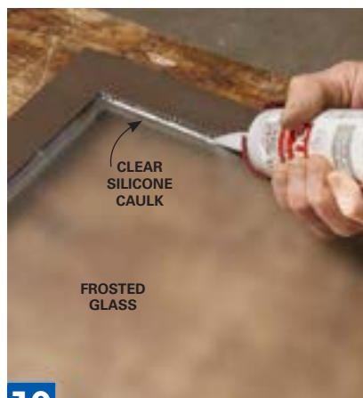
10 Install the glass. After the paint dries, set the glass panels in the rabbet and apply a small, neat bead of clear silicone around the perimeter. Let the silicone cure overnight before mounting the doors.
