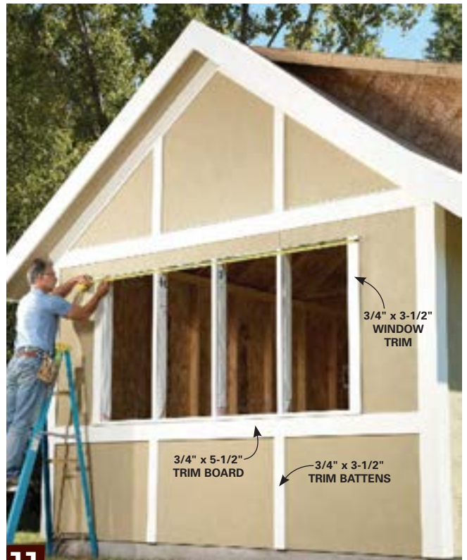
11 Trim with PVC boards. Cut and nail the PVC trim just like wood. Use a sharp carbide blade on a miter saw to cut it, and stainless steel or hot-dipped galvanized nails to fasten the trim to the framing. Battens cover all the siding seams.
