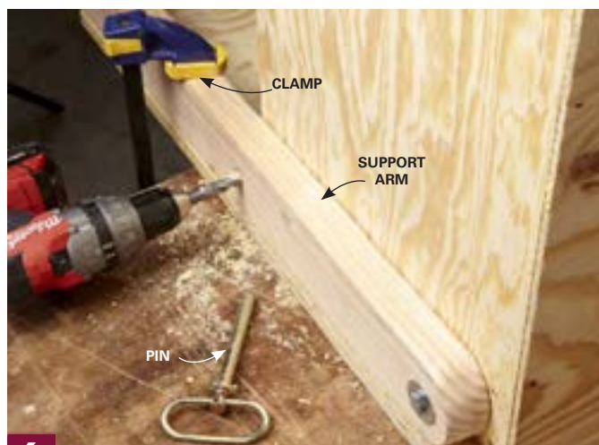
6 Drill the pin hole. Make sure the folding top is clamped securely to the support arm before you drill a hole for the hitch pin. When drilling a hole this big, it's easier to start with a pilot hole about half the size.
