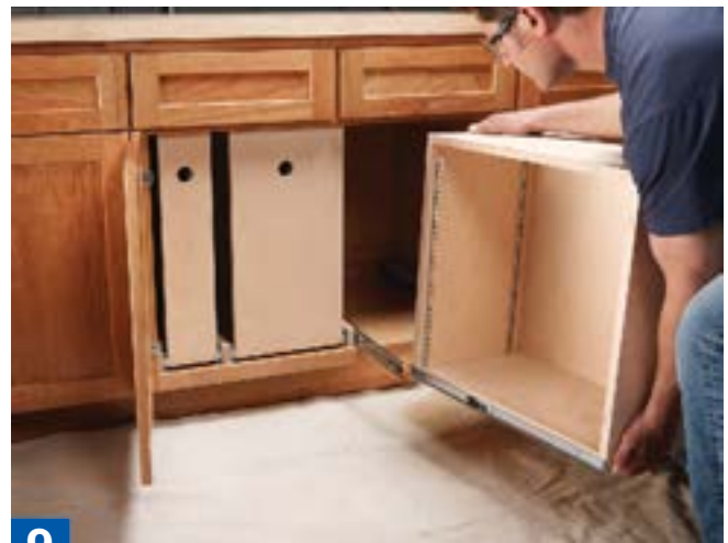
9 Slip the box-mounted slides into the cleat slides and push the box all the way in to fully engage the slides.
