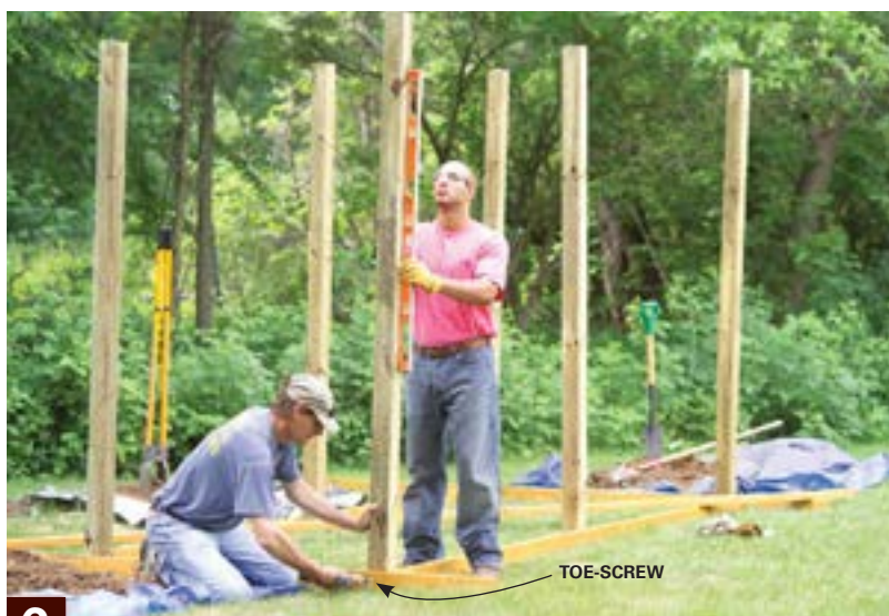
2 Drop the posts into the holes, position them using the template, plumb them and screw them into place. Fill the holes with concrete.
