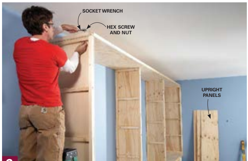
3 Set the top on the uprights and bolt it to them. Also bolt the uprights to the base. Then nail plywood panels to the uprights to enclose the framing.
