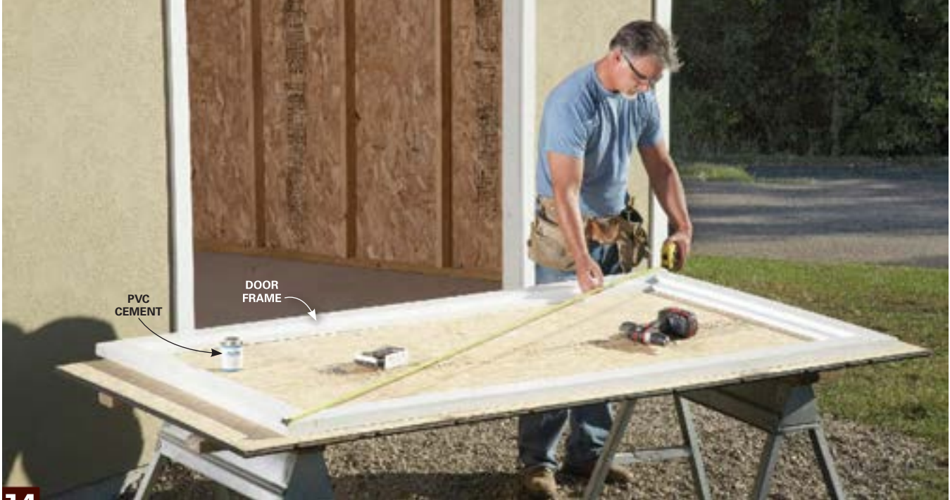
14 Build the doors. Build the doors from PVC boards and fiber cement panels. Weld the overlapping PVC frame pieces with special
