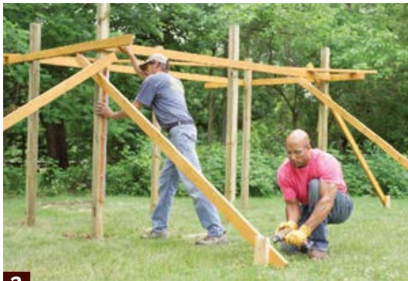
3 Slide the template up 5 ft. and level it, screwing it to the posts. Recheck the posts for plumb and brace the assembly. Let the concrete harden overnight.
