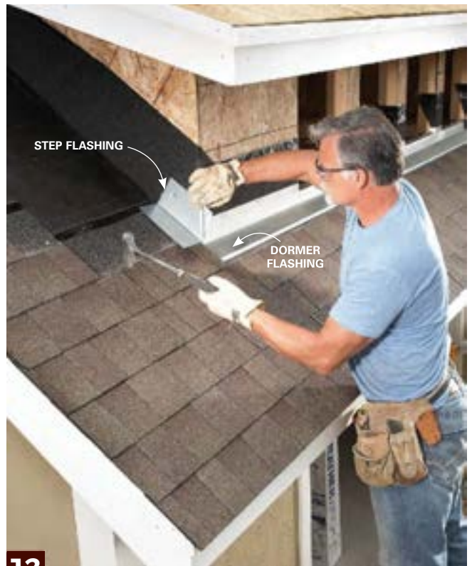
13 Roof before siding the dormer. Shingle the roof of the main structure before you side the dormer. This allows the siding to go over the top of the metal flashings.
