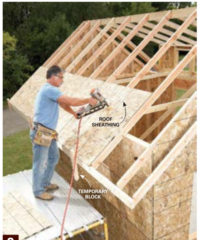
8 Sheathe the roof. Nail temporary blocks to the subfascia to hold the first row of sheathing in place. Space the sheets 1/8 in. apart. If you don't leave gaps, you might get ridges that show through the shingles when the sheathing swells.
