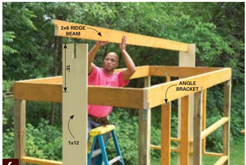
6 Cut a slot, then center and nail a 1x12 siding board to each end wall. Then drop the ridge board into the slots and center it.
