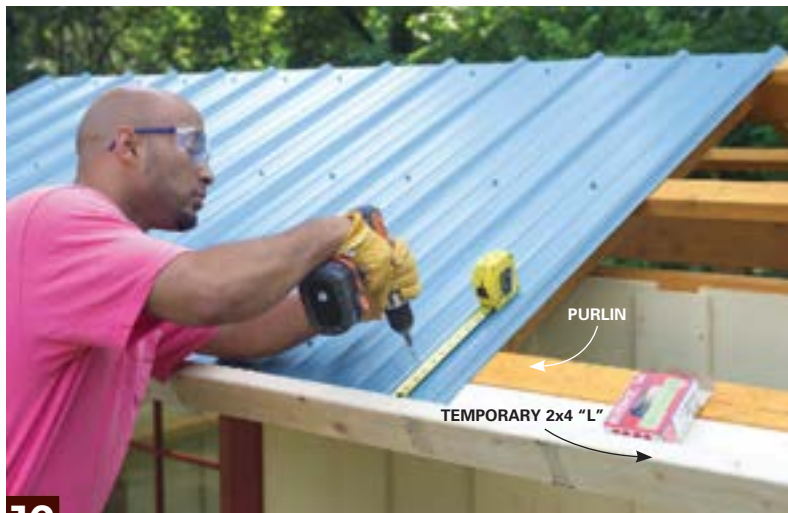
12 Screw a 2x4 "L" to the rafter tails tight against the bottom purlin. Then rest the roof panels against it and screw the panels to the purlin.
