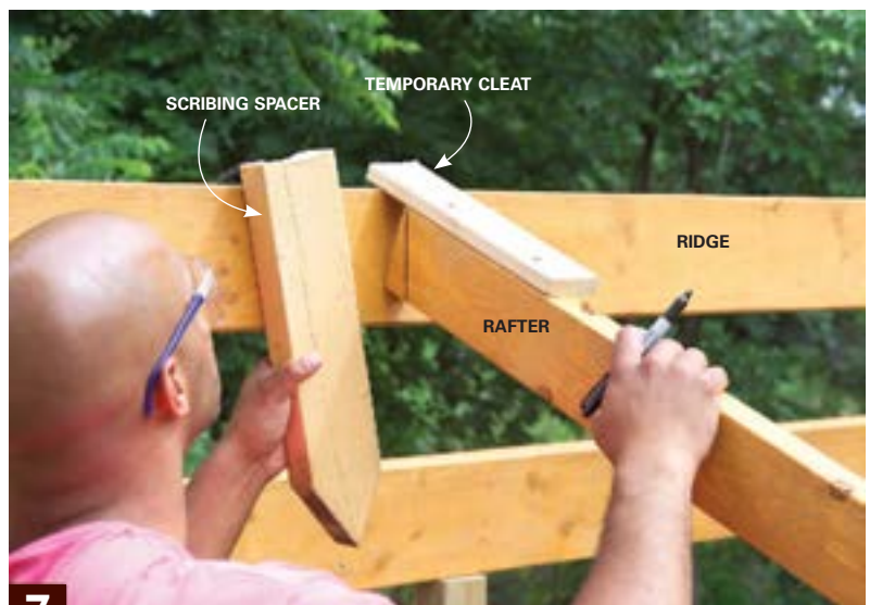
7 Scribe the ridge angle cut on one of the rafters and cut it to length. Use it as a pattern to mark the other rafters.
