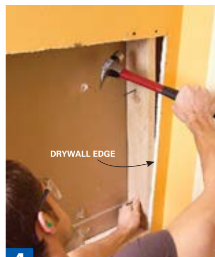
4 Cut and tap in vertical backing flush with the drywall edge, then toe-screw it to the blocking.
