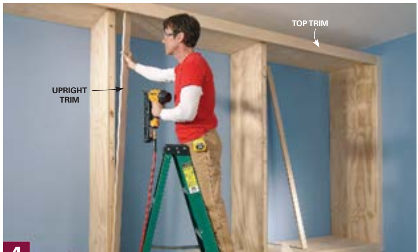
4 Dress up the front edges of the base and uprights by nailing on trim boards. The top trim overhangs the top to hide the door track.
