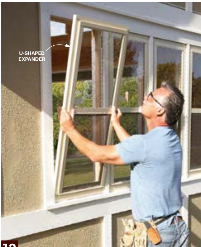
12 Screw in the aluminum windows. Apply a small bead of caulk to the stops and press the window against them. Slide the expanders tight to the opening and screw through them into the stops.
