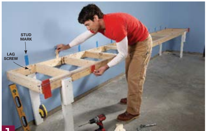
1 Support the base frame with temporary legs and screw it to wall studs. Use a string line and shims to make sure the front edge is perfectly straight.
