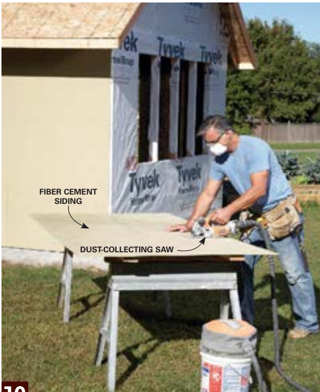
10 Cut and hang the siding. Lay 2x4s over sawhorses to support the sheets while you cut. If you don't have a special saw, use your regular circular saw with a carbide blade. Fiber cement is tough on blades, so don't waste money on an expensive blade. Nail the siding to the studs.
