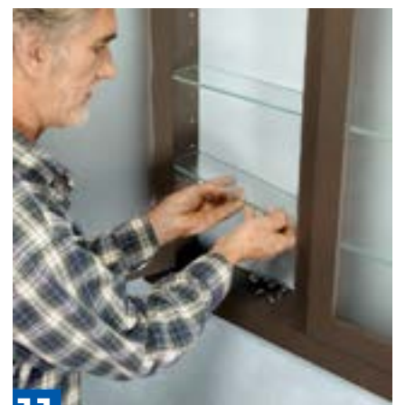
11 Install the cabinet and shelves. Set the cabinet in the wall and level it. Then attach it with screws driven into the shelf support holes. Finish the project by clipping the doors to the hinge plates and installing the glass shelves. Use the hinge adjusting screws to adjust the doors until the space between them and the cabinet is even.
