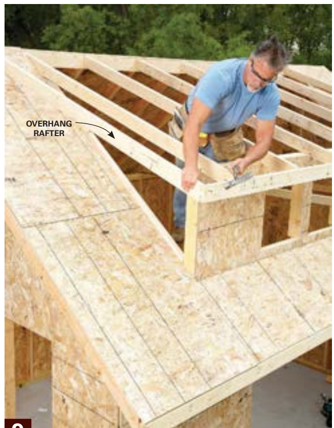
9 Finish the dormer framing. Complete the sheathing on the main roof before adding the overhang rafter so you don't have to notch the sheathing to fit around the rafter.
