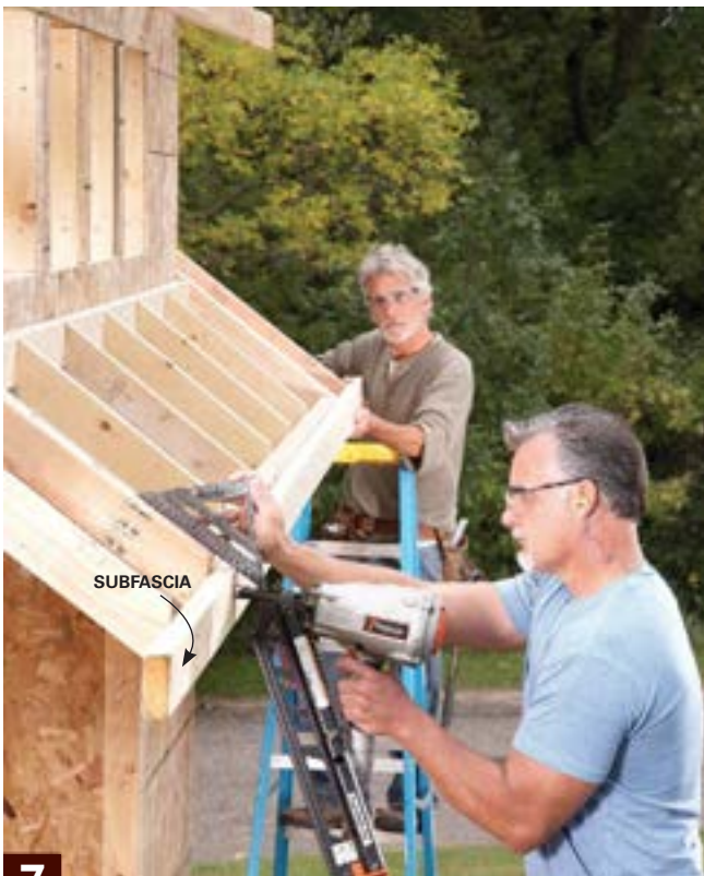
7 Nail on the subfascia boards. Align the top of the 2x4 subfascias with the top of the rafters. Start nailing at one end and have a helper at the other end raise and lower the board to line it up while you nail it.
