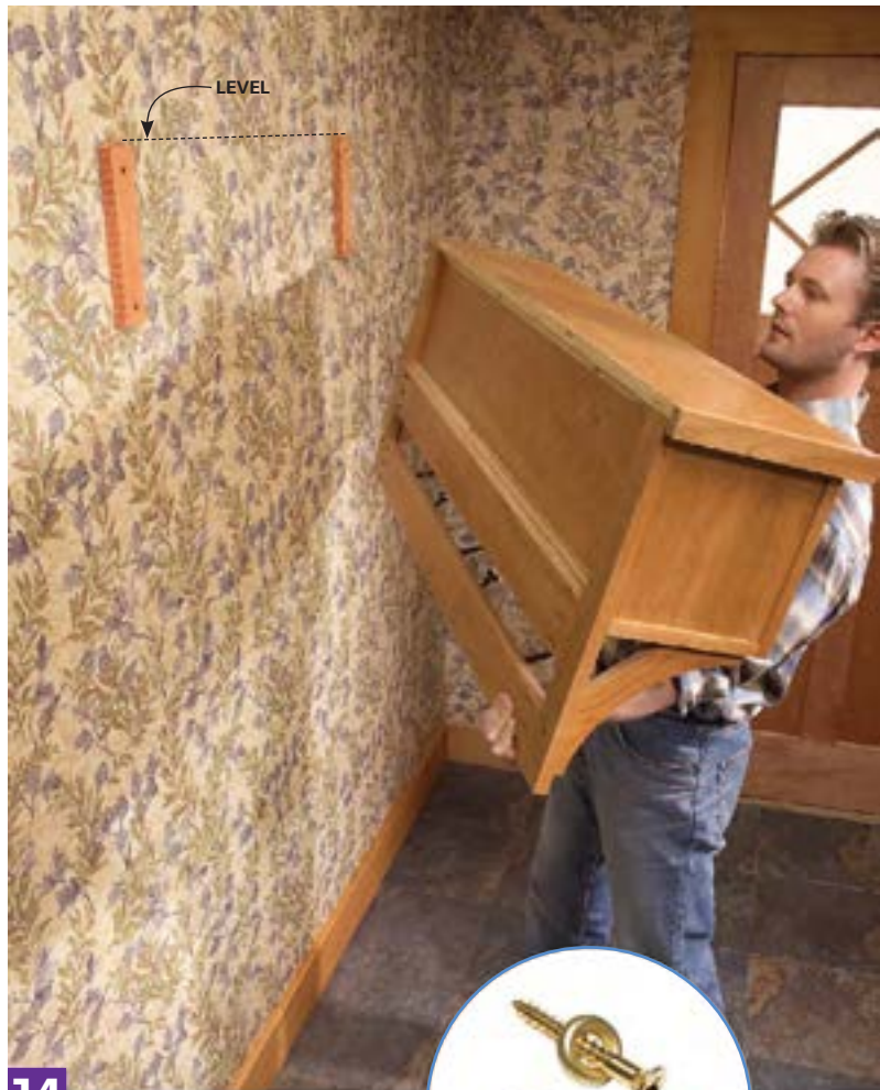
14 Level and screw 2-in. x 8-in. cleats to wall studs. Set the shelf on the cleats and screw through the back of the shelf into the cleats using 1-1/2-in. brass screws and finish washers.
