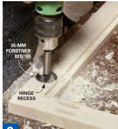
8 Drill concealed-hinge mounting holes. Mark the hinge hole locations. Use an awl or nail to make a starting point for the Forstner bit. Drill recesses for the hinges in both doors.
