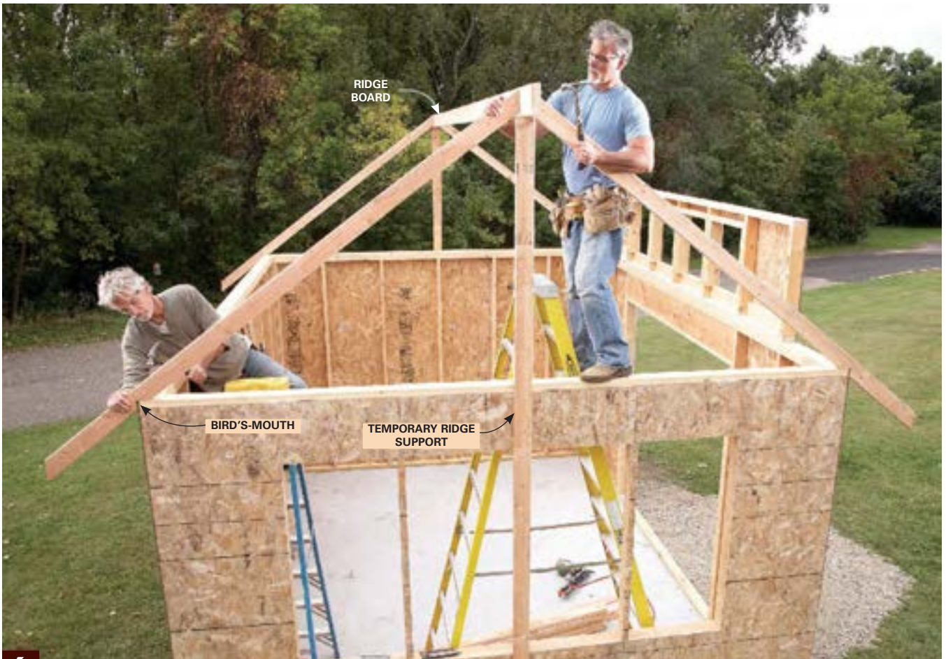
6 Frame the roof. Mark the rafter locations on the ridge board and prop it up with temporary supports. Nail the rafters to the ridge
