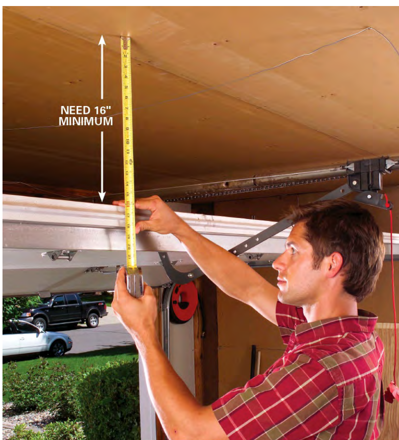
1 Measure from the ceiling to the top of the raised garage door. Subtract 1 in. to determine the height of the side 2x4s.
