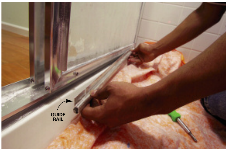
1 Unscrew the guide at the lower edge of the sliding door. Protect the shower or tub from scratches with a drop cloth.
