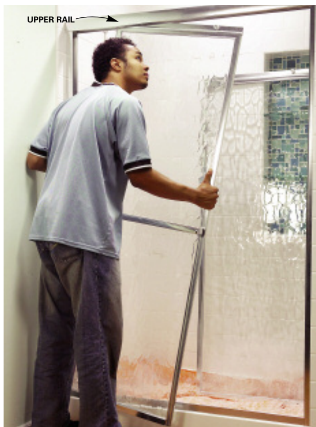
2 Lift the door out of its track inside the upper rail. Tilt each door in or out to remove it. Wipe both tracks clean.
