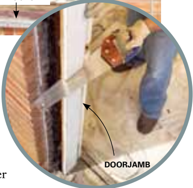
4 Cut completely through the side jamb with a handsaw. Pry the jambs loose and pull them out of the opening.
