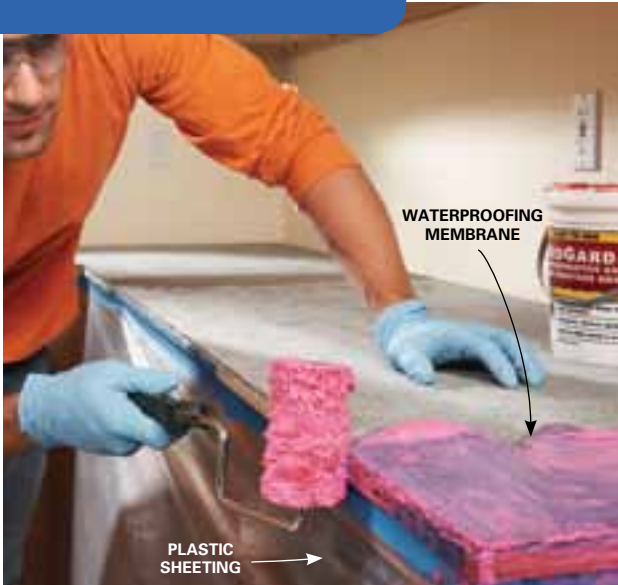
1 Protect the tile base against water damage with a coat of waterproofing membrane.
