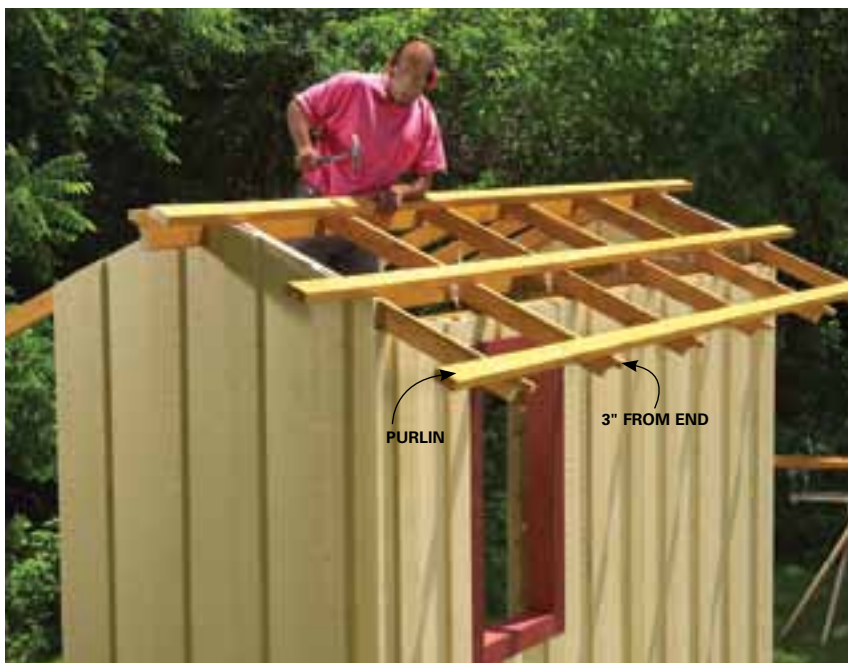
11 Cut the purlins to length, then center and nail them to each rafter with two 16d nails.
