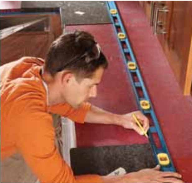
5 Draw a baseline from the inside corner tiles to the end tiles. Use this line as a guide as you set the front row of tiles.
