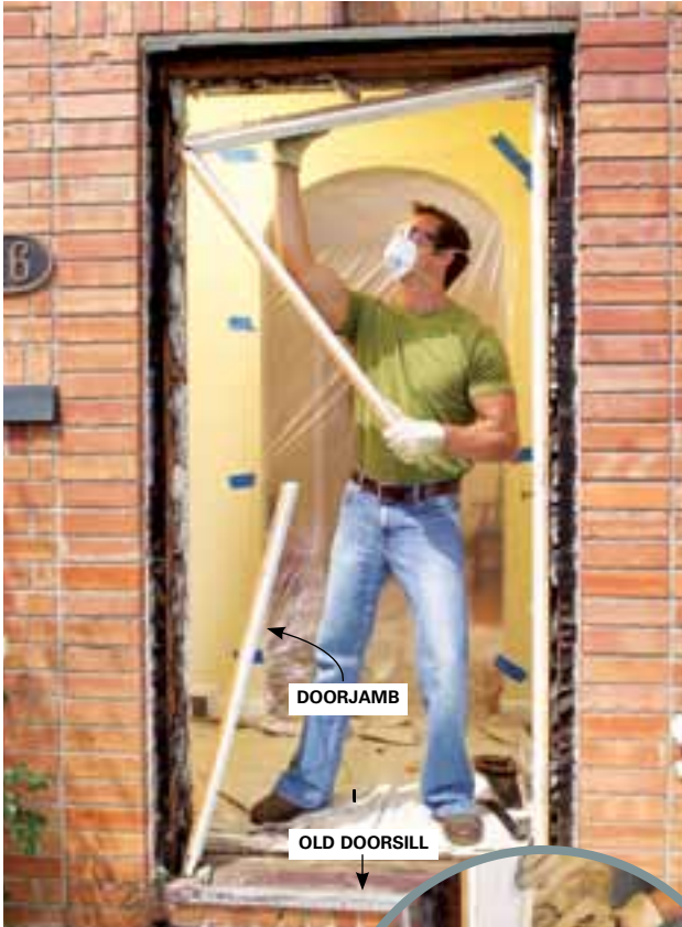
4 Cut completely through the side jamb with a handsaw. Pry the jambs loose and pull them out of the opening.
