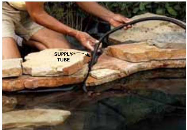
4 Surround the pond with stones. Leave a gap between stones so you can remove the waterfall supply tube if necessary. Do the same for the pump's power cord.
