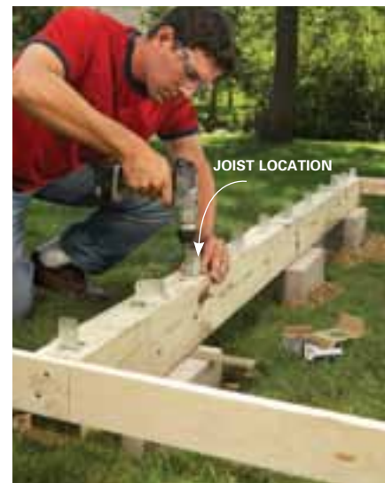
3 Screw on angle brackets at each joist location instead of toenailing, which can split and weaken the joists and knock the beam out of square.
