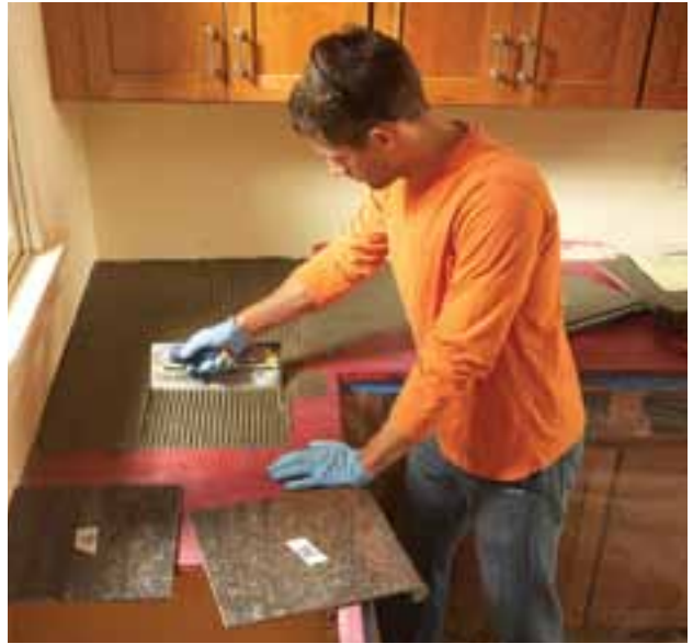
6 Work in small sections, spreading just enough thin-set to set eight tiles. That gives you plenty of time to set and adjust tiles before the thin-set becomes too stiff.
