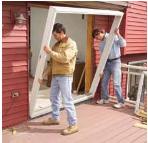
8 Assemble the frame following the manufacturer's instructions. Apply two beads of silicone caulk along the length of the threshold and tip the frame into the opening.
