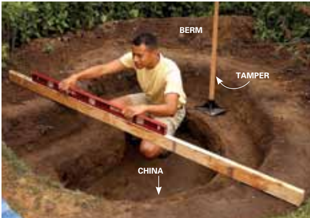
1 Dig the pond hole. To form a level rim, scrape away soil on the high side and build a bank on the low side. Compact built-up soil with a tamper.
