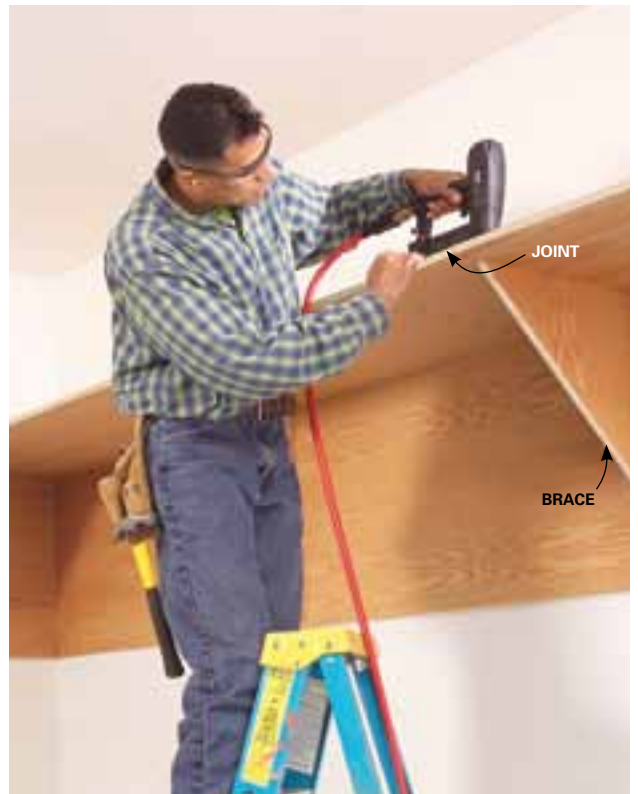
6 Nail the shelves to the apron and to the braces with 2-in. nails spaced every 8 in. Make sure joints meet at the center of the 3/4-in. braces.
