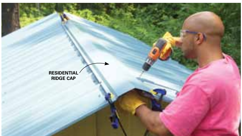
13 Cut both ridge caps to length, then center and clamp them into place. Screw them to every third rib.
