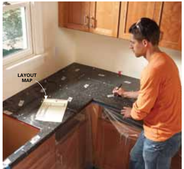
4 Number the tiles and sketch a layout map after the dry run. Remove the tiles and use the map to put each tile back in the correct order later.
