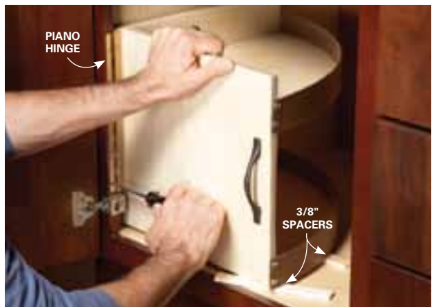
2 Hang it on a hinge. Raise the shelf with spacers and align the shelf back with the inside edge of the face frame. Screw the piano hinge to the shelf back, then to the cabinet. You may have to notch the shelf back to clear the door hinge.
