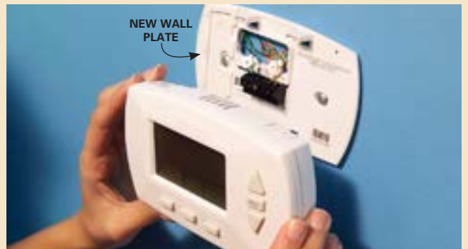
4 Install the batteries, program the thermostat and snap it onto the wall plate.
