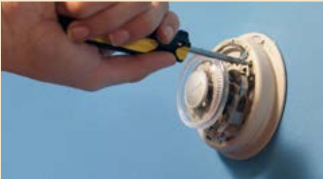
1 Pull off the cover ring and remove the screws that fasten the thermostat to the wall plate.
