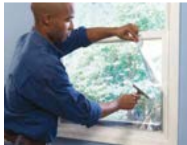
Window film can be installed in about 30 minutes. The hazy appearance will disappear after 10 days.
