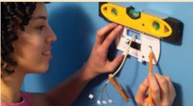
3 Mark the new screw locations, drive in wall anchors and screw the mounting plate to the wall. Connect the wires.
